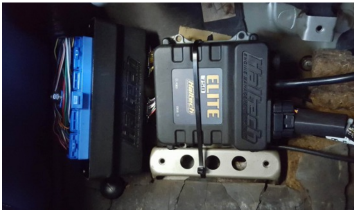
Figure 3 - Installation of Haltech products
